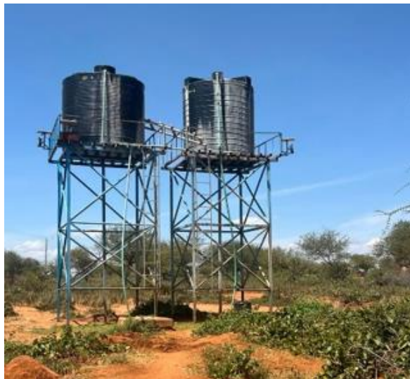
Figure 3 Water storage tanks on site
