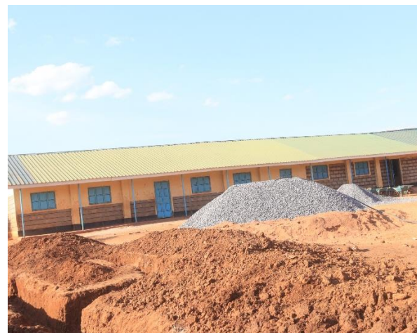
Figure 3 Lekurruki Primary School on site
