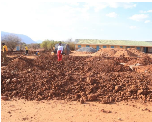
Figure 2 Expansion efforts on site
