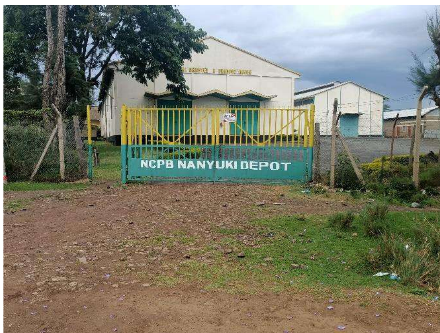
Plate 8-2: Grain Warehouses at Nanyuki and Ol Moran
