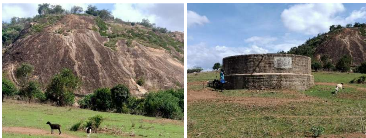
Plate 9-8: A Rock Catchment and Community Storage Tank
