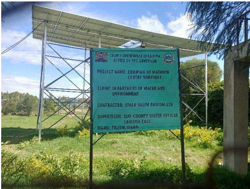
Plate 9-9: A Solar Powered Borehole in Matanya and Water Storage Tank within Nanyuki Township
