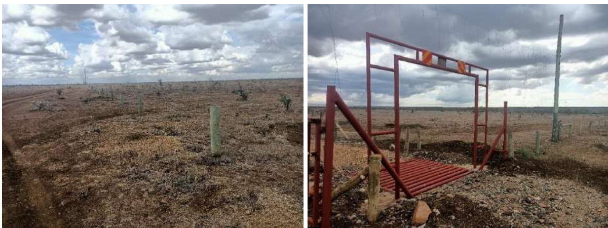
Plate 4-13: Restrictive Low-hanging Fencing and Obstructive Infrastructure on a Movement Corridor
