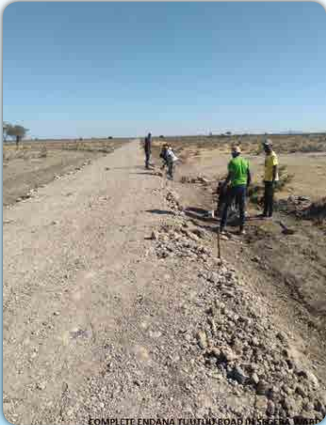
COMPLETE ENDANA TUUTU ROAD IN SEGERA WARD
