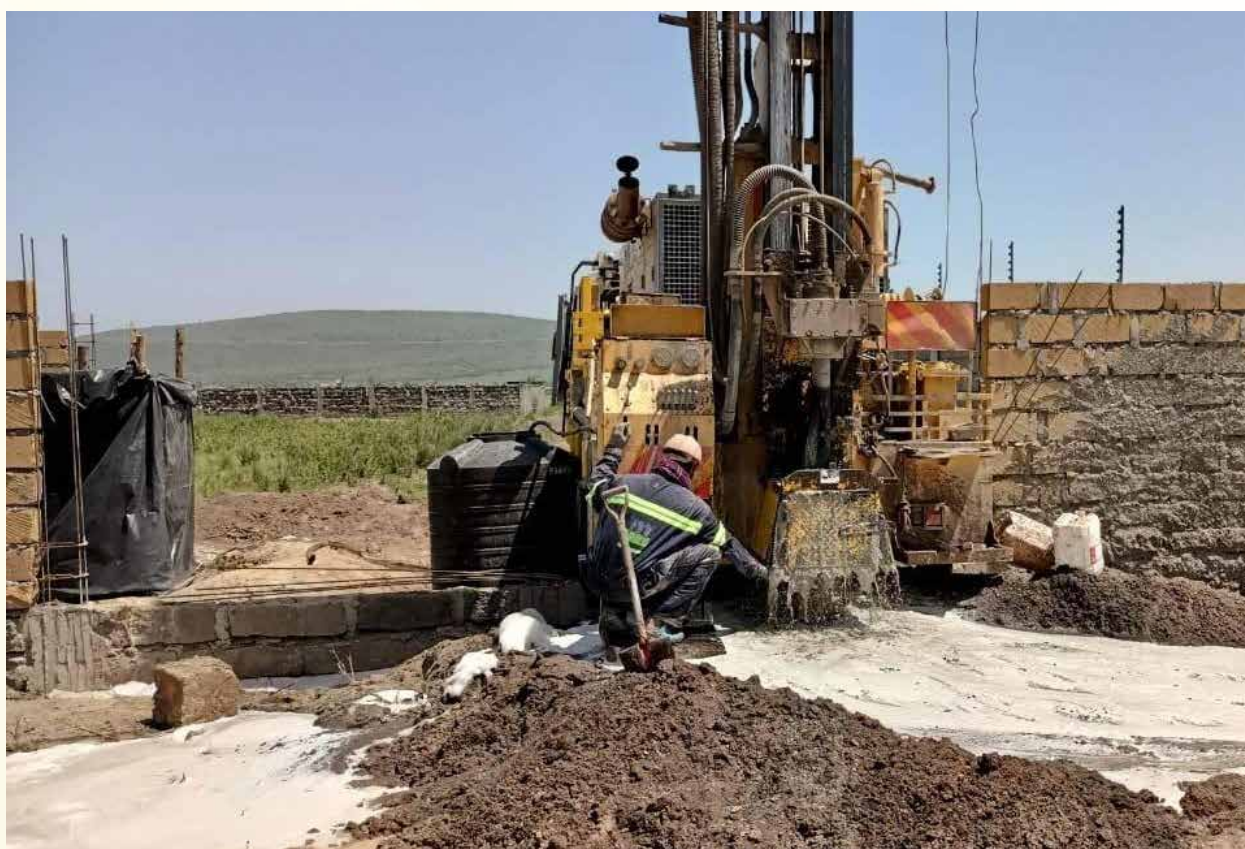
Borehole drilling in Laikipia County
