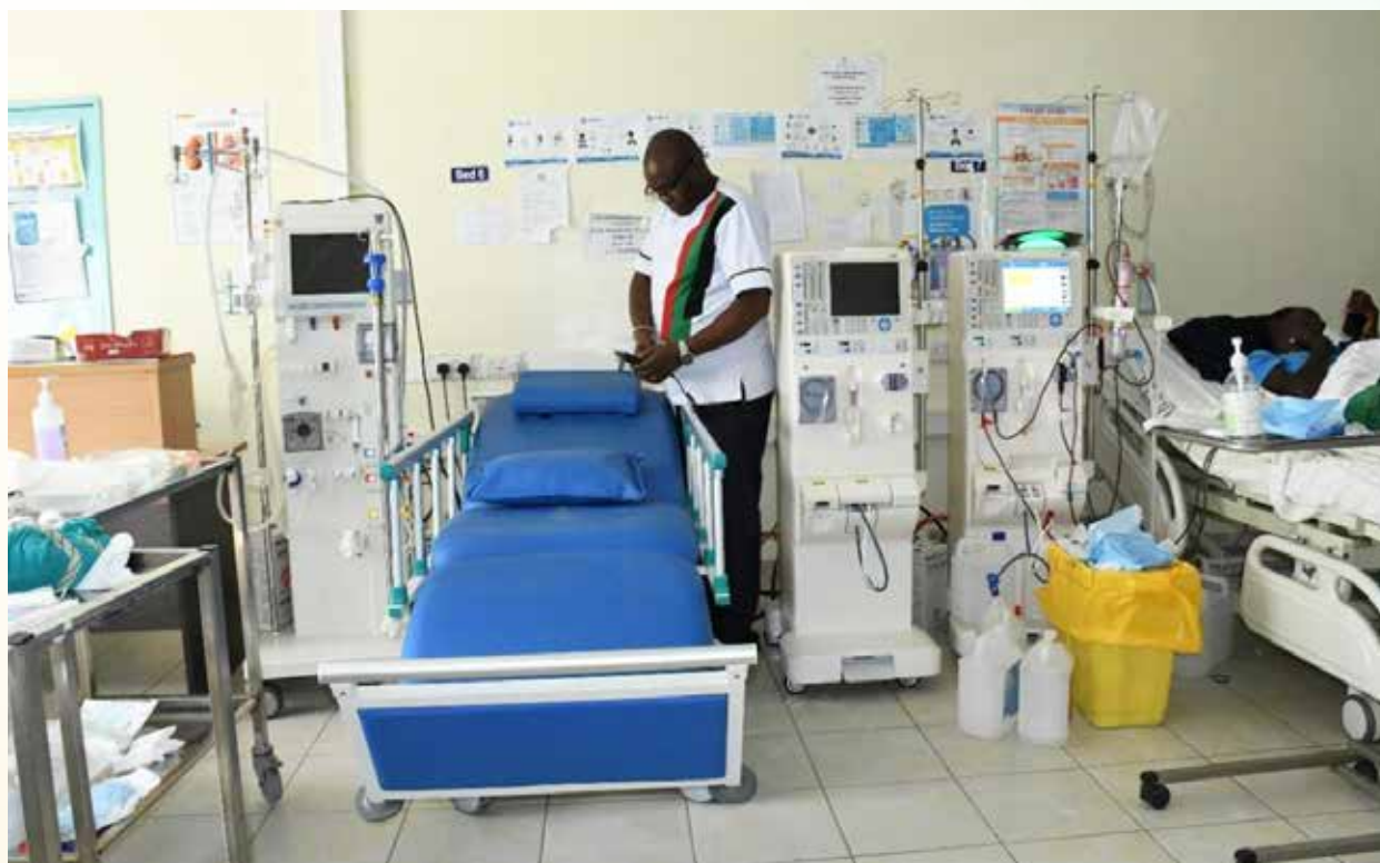
It's now systems go- the additional renal dialysis beds now fully installed, and ready to go
