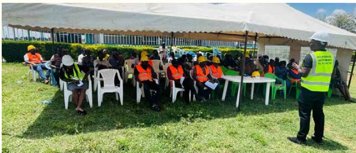
Ground breaking for the construction of a male ward at Rumuruti Sub-County Hospital (LHS Rumuruti)
