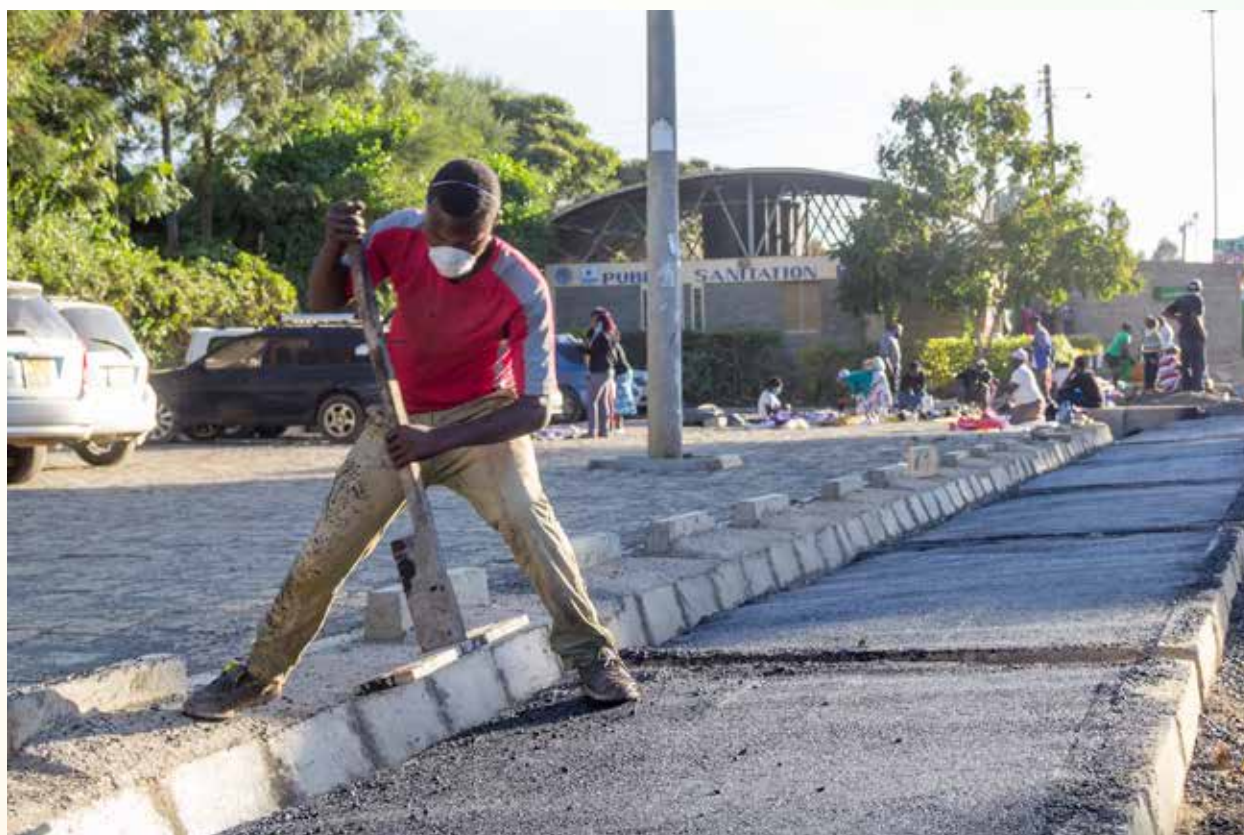
Road works in progress
