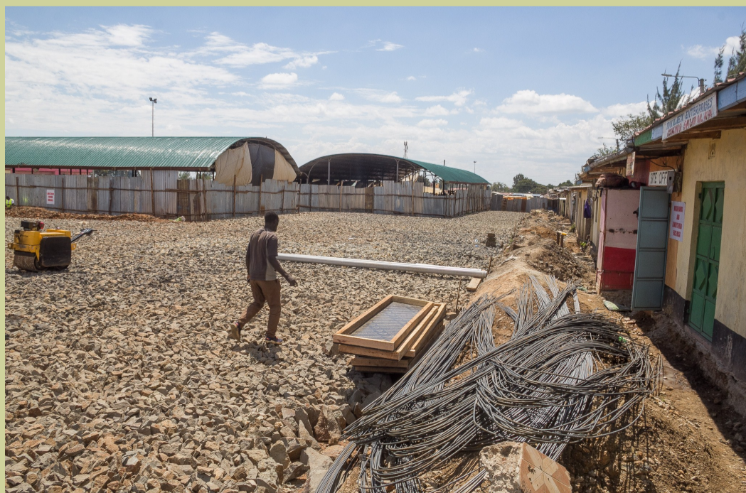
Construction work at Nanyuki Old Open Air Market promote business.
