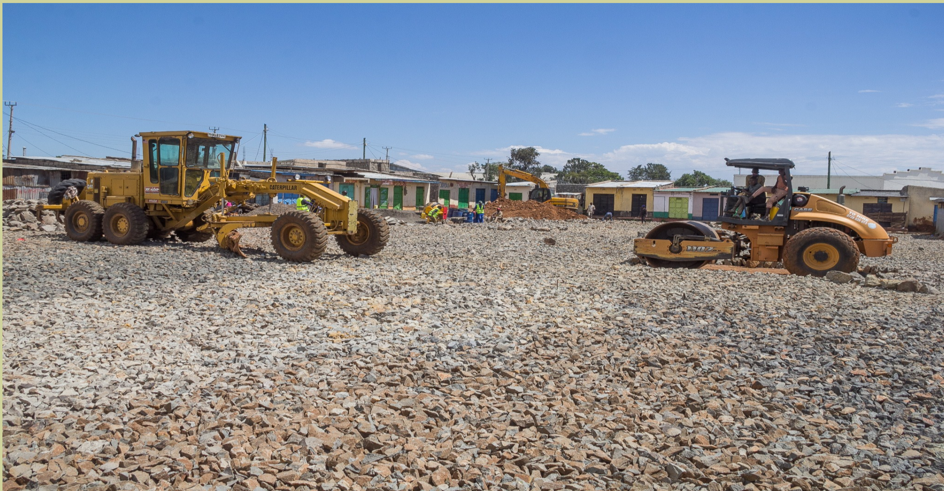
Construction work at Nanyuki Open Air Market promote business
