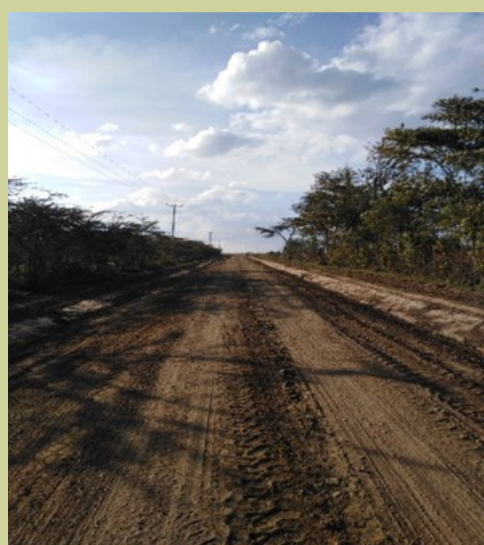
Pefa- Kiमारiga road grading
