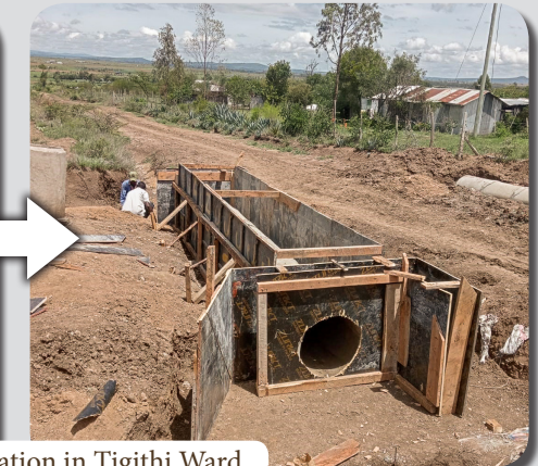
Culvert installation in Tigithi Ward
