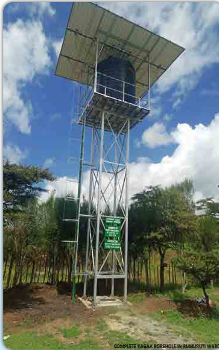
COMPLETE KAGAA BOREHOLE IN RUMURUTI WARD
