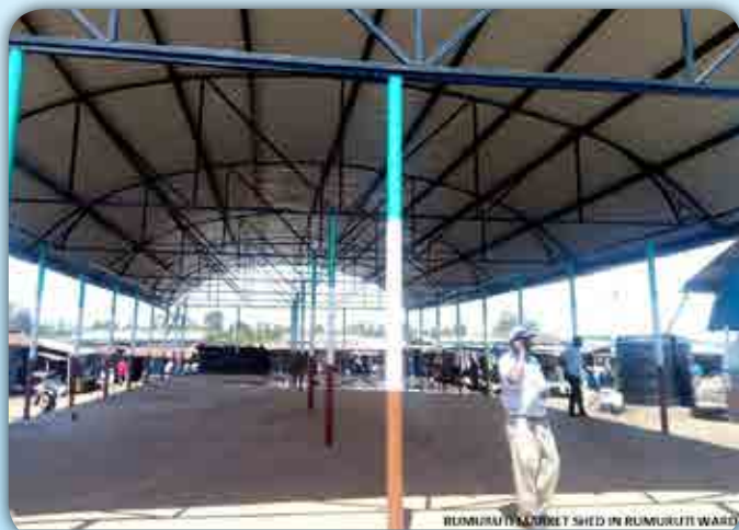
RUMURUTI MARKET SHED IN RUMURUTI WARD
