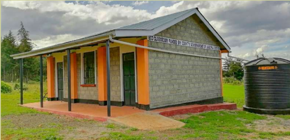
A newly-buit ECDE classroom by the county Government in Igwamiti Ward
