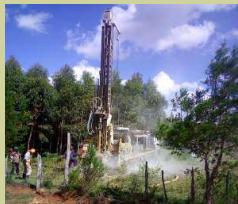
Drilling of Gatitu borehole
