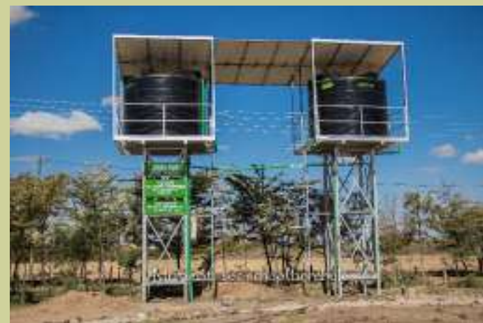
Muramati primary school borehole
