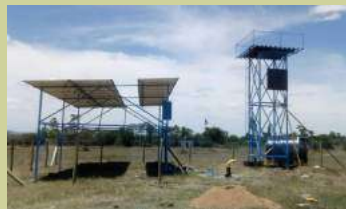
Matanya health centre and community borehole in Tigithi Ward (ongoing)
