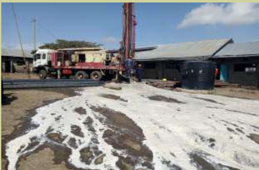
Drilling of Mwiyo Primary School Borehole- Tigithi Ward
