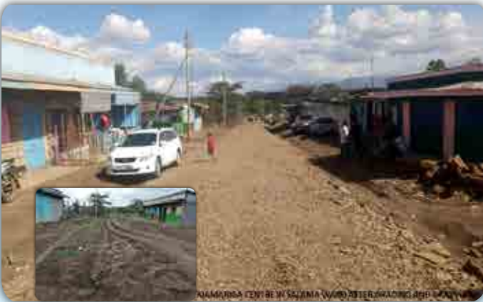
ROAD IMPROVEMENT PROJECT IN SALAMA WARD
