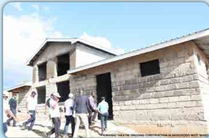
KIMANDO THEATRE ONGOING CONSTRUCTION IN MUKOGONDO WEST WARD
