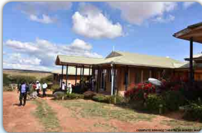
COMPLETED KIMANDO THEATRE IN MUKOGONDO WEST WARD
