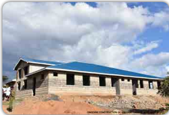
ONGOING CONSTRUCTION OF KIMANDO
