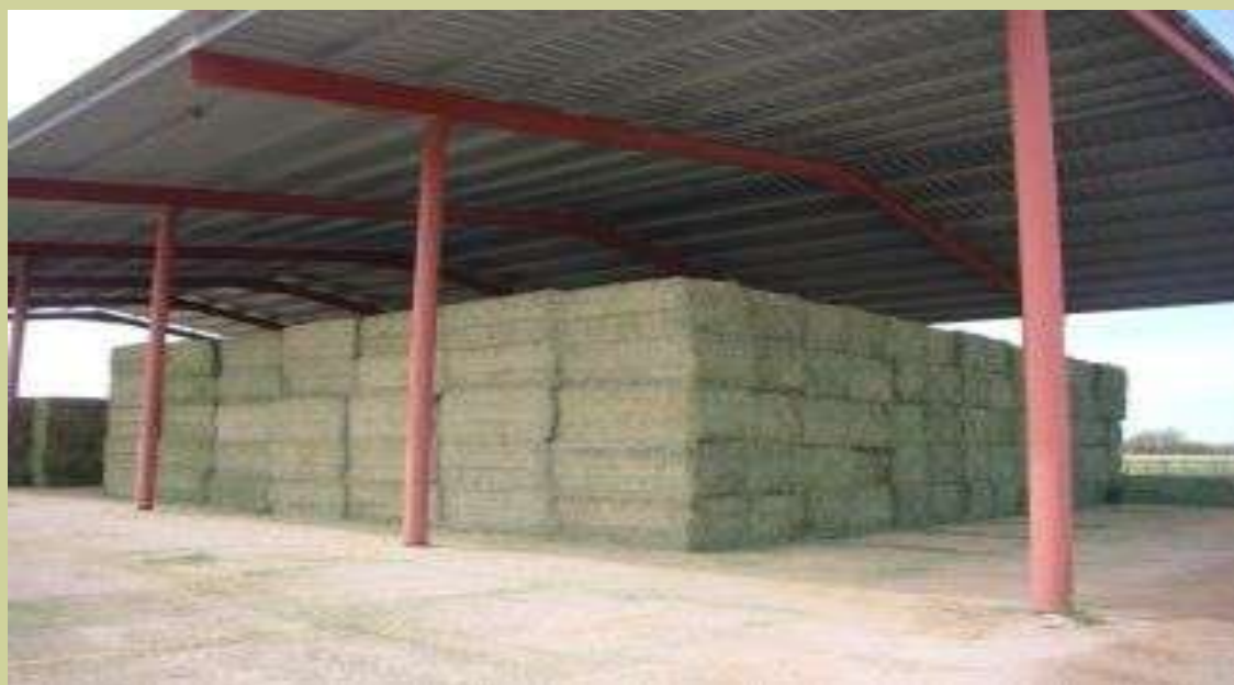
A modern hay shed at Matanya with a capacity to store 25,000 bales of hay
