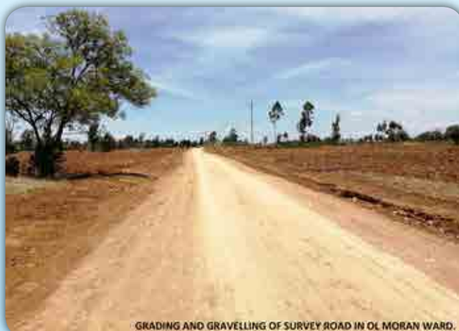
GRADING AND GRAVELLING OF SURVEY ROAD IN OL MORAN WARD.
