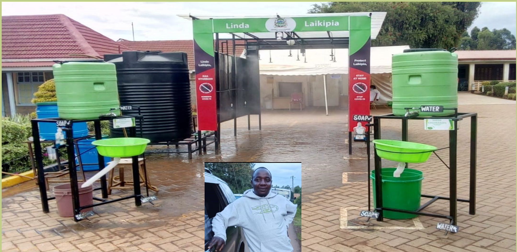
Two sets of contact-free safe hand-washing facilities at the Nyahururu County Referral Hospital. (inset) Joseph Nderitu
