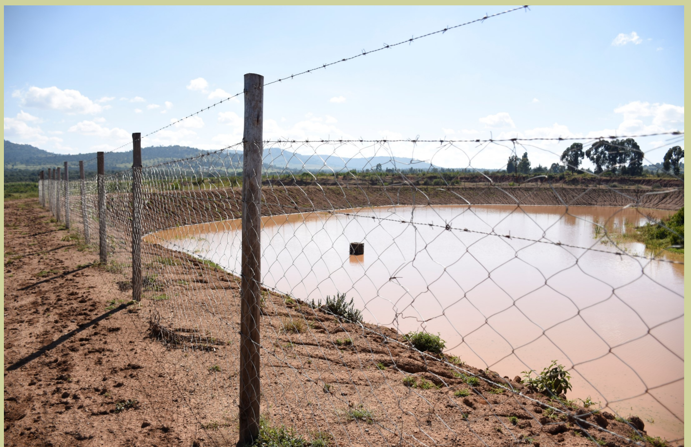
Matwiku dam that has been done through the KCSAP
