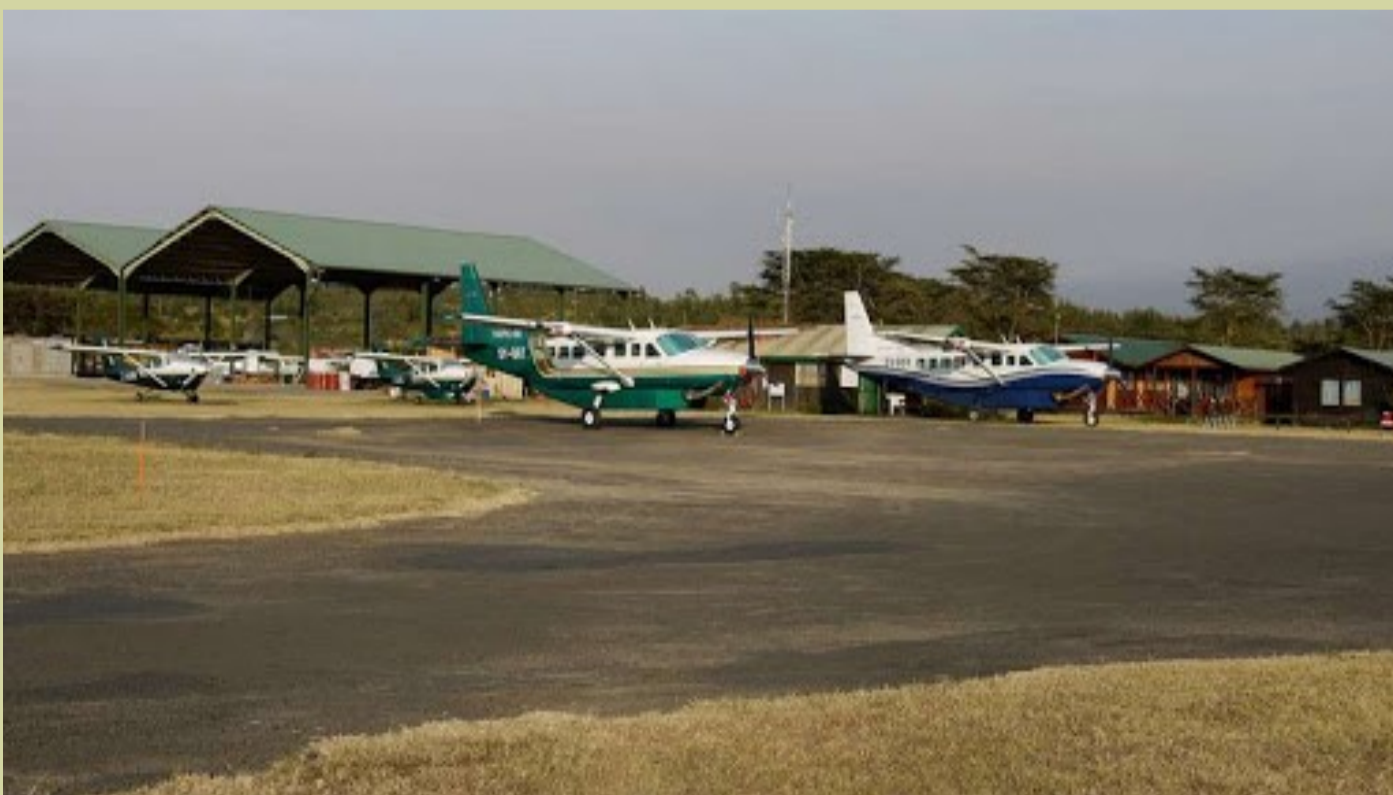
The busy Nanyuki Civil Airstrip which is undergoing an extreme makeover plays a critical part in Laikipia's tourism
