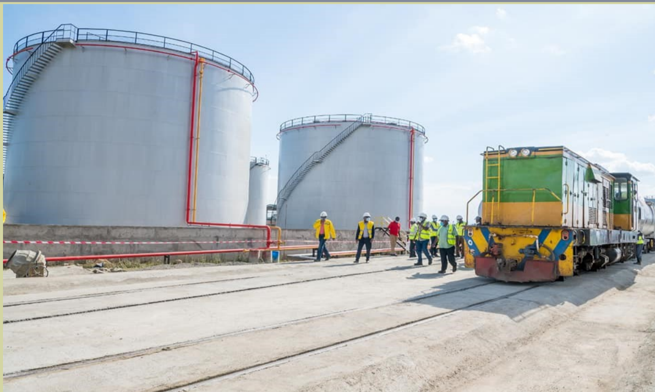
The new 11.5 million litre Vivo Energy fuel depot in Nanyuki
