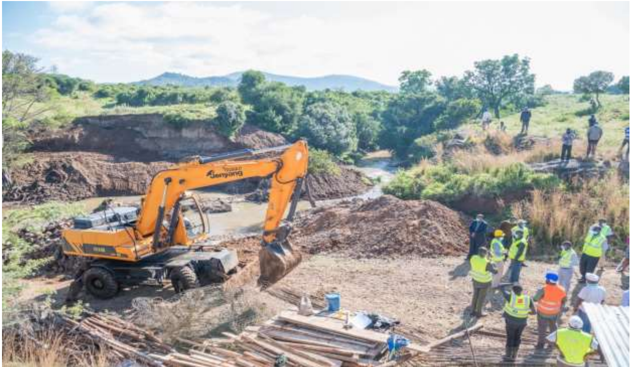
Bridge construction- Muramati
