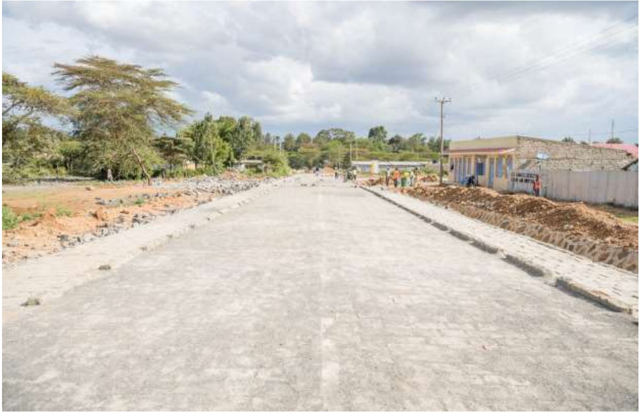
Cobblestone works- Rumuruti town
