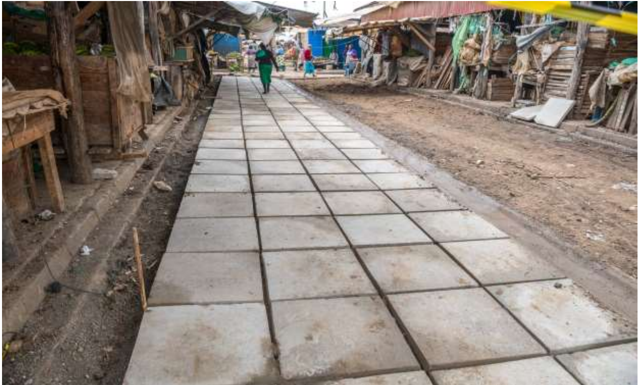
Marikiti market rehabilitation- Nanyuki ward
